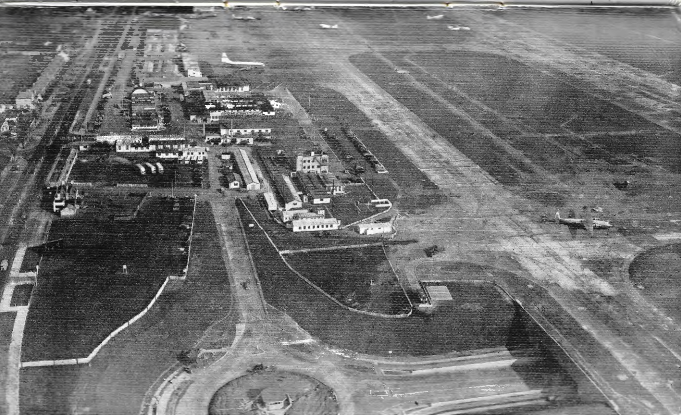
Oblique aerial view of temporary terminal area
