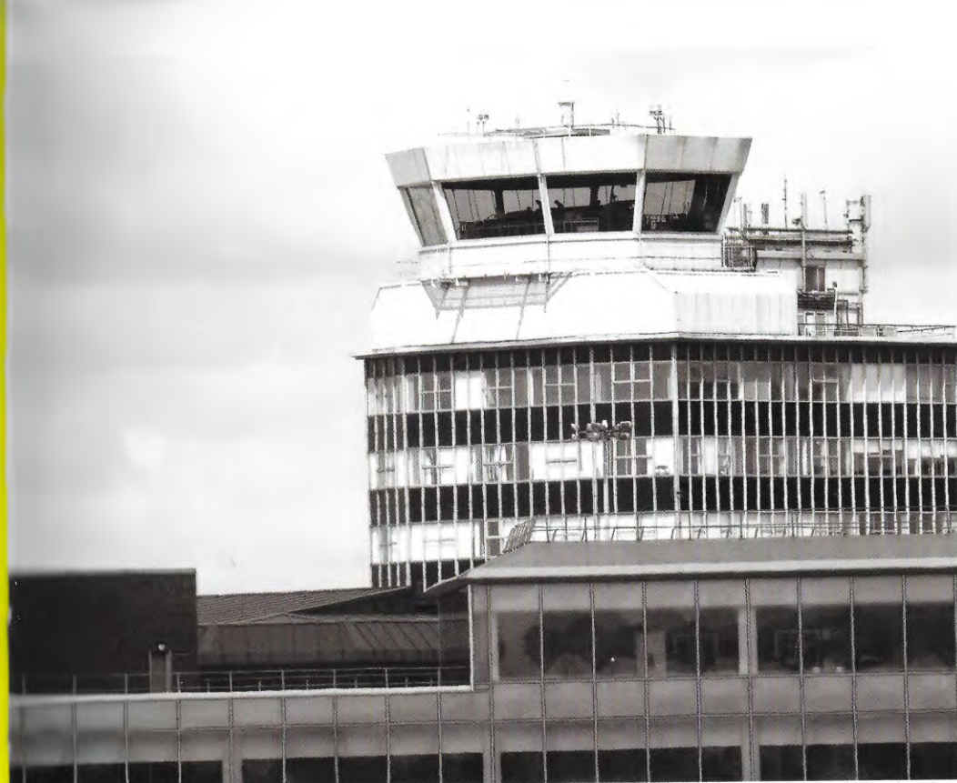
Manchester Tower, within which is Manchester Area Control Centre
