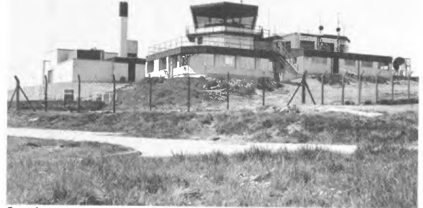
Control tower and meteorological office
