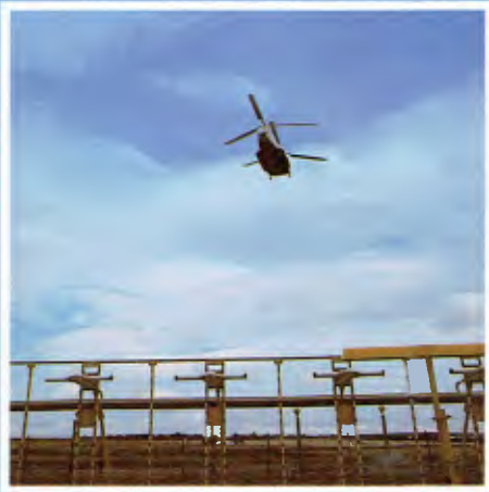
The localiser aerial
