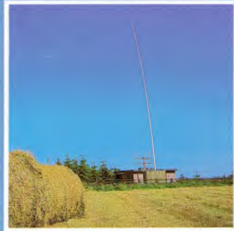
The non-directional beacon
